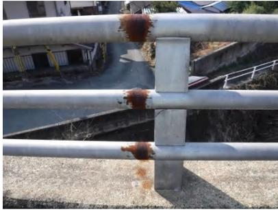
Fig.3 Only welds are rusted
